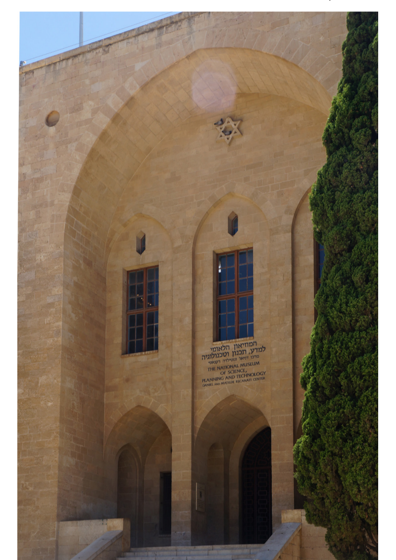
Fig. 2, 3, 4, 5: Detailed Fotos: pointed arches, cupolas, ventilation openings over the windows, crenellations
