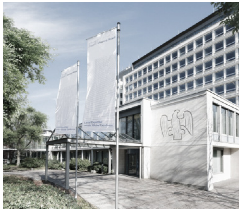
Fig. 3 - External view of the entrance
