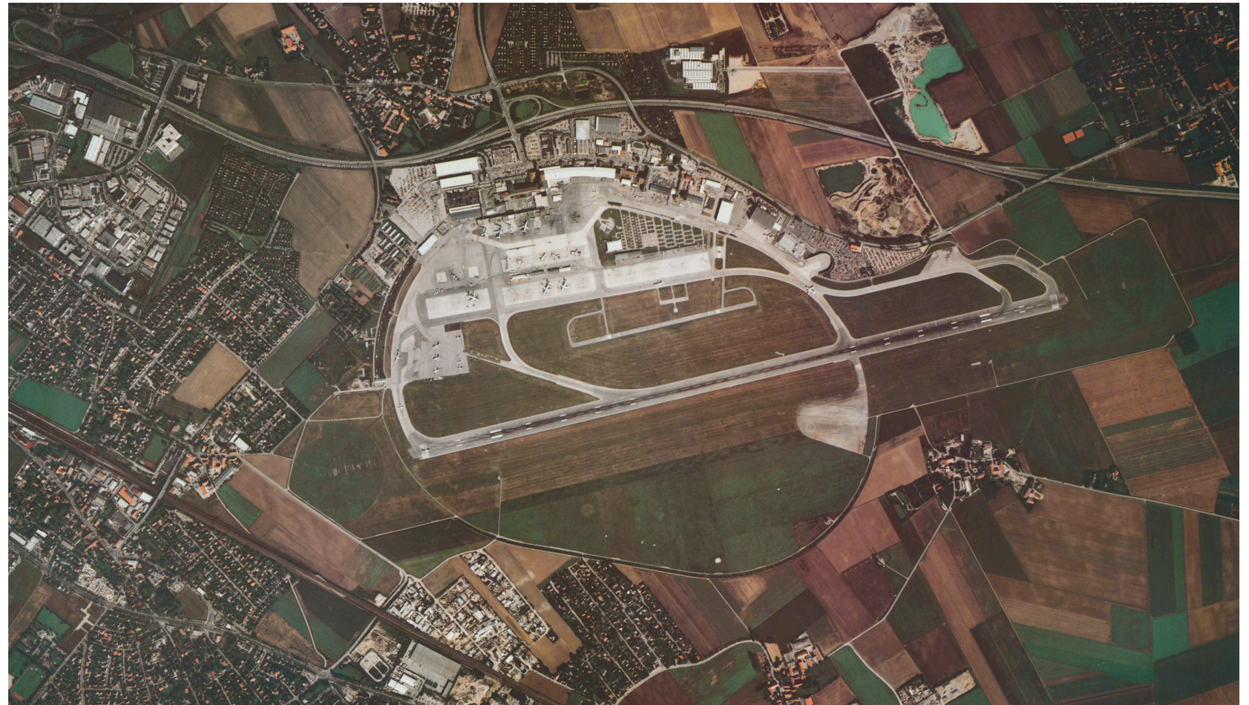
Fig 1: Aerial view of the airport
