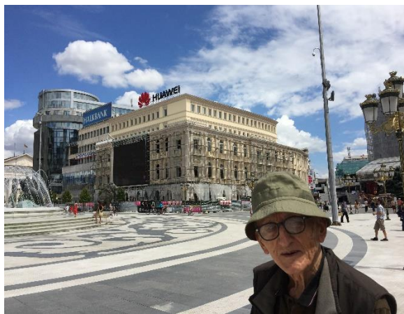
Fig. 5: Slavko Brezoski standing in front of his newly remodeled building.
