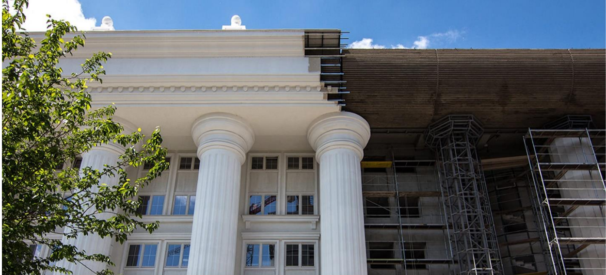
Fig. 1: Part of Skopje's telecommunications center receiving a baroque treatment.
