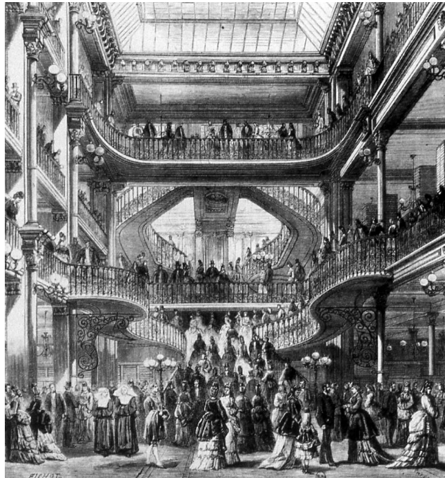
fig #1: main staircase of Le Bon Marché , 1982
