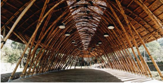
D.Z. Architects & Associates Butterfly Bamboo Pavillons Nantou County, Taiwan 2019 © Chih-Chieh YU and Boo-Him LO
